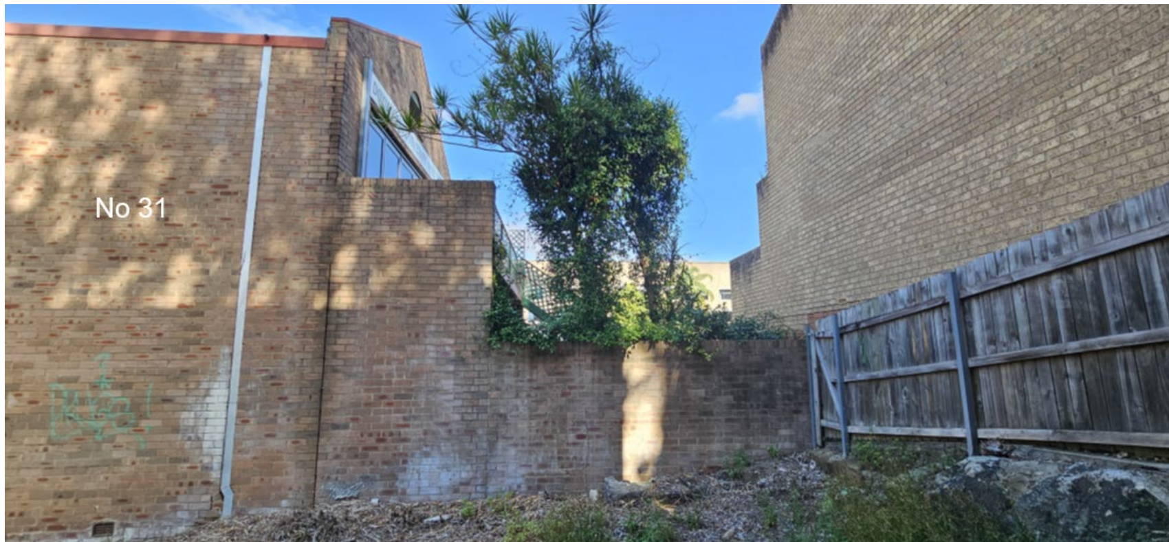
adjoining building to south - No 31
